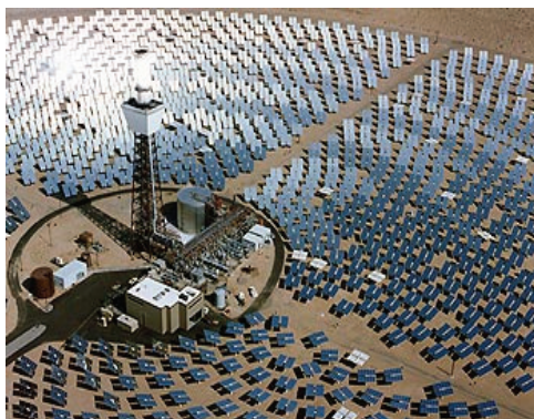
Fig. 5. Heliostat field with a central tower Solar Two, in Barstow, California
